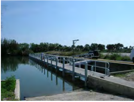
Improved Bair's Cove Boat Ramp Photo by Dorn Whitmore Supervisory Ranger
